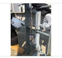
5. The nuts on the tensioner can now be tightened against the turnbuckle, locking it in place. All system components should be checked, ensuring all are secure and nothing has been missed.
