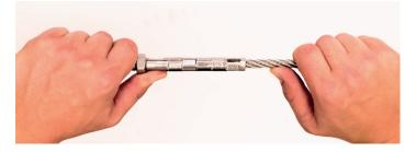
15. The termination has now been fully crimped and can be connected to the post by removing the pin/bolt and securing to the start/end post.
