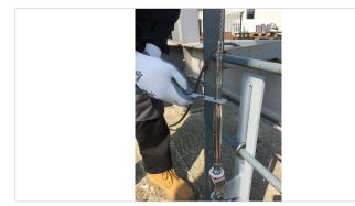
3. By holding the crimped barrel and line in one hand the turnbuckle/central barrel of the tensioner can be turned, tensioning the line with the other hand.
