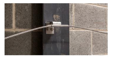
3. Working from an anchor point along the line, take up the tension to remove as much sag as possible. Clamp off at the last component.
