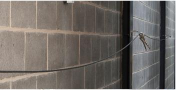
2. To gain the most accurate measurement it is advised to swage/crimp the end termination and fix to the end anchor points. If the end component is a line tensioner, ensure the tensioner is fully wound out prior to crimping. See section on crimping/swaging for more details.
