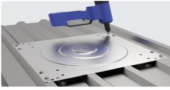
6. Turn bolt onto female boss in base plate by hand firstly then to the desired tightness of 20Nm with the 19mm spanner until Anchor Point is seated correctly.
