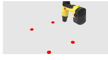
4. Ensure you have the correct stud length for the total build up depth, embedment into the substrate and enough protruding from the opening to fit a nut and washer.
