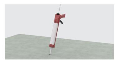
4. Once the resin is prepared squeeze resin through hole into substrate, slowly retracting the nozzle as the hole fills until 2/3 full.
