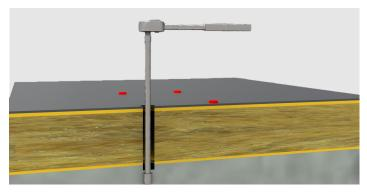
7. Turn studding into screw head of each fixing ensuring the correct stud length is used to allow enough to protrude from the opening to fit a nut and washer.
