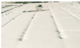
Cold bridging via all-carbon steel fasteners
