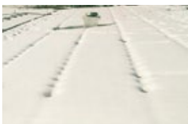
Cold bridging via all-carbon steel fasteners
